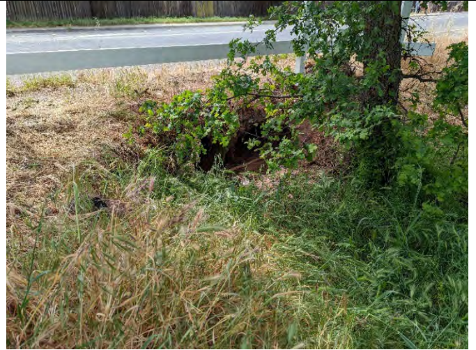
Culvert at the southeastern corner of the BSA, facing south.
