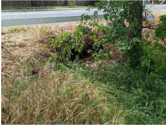
P01 – Culvert looking southwest
