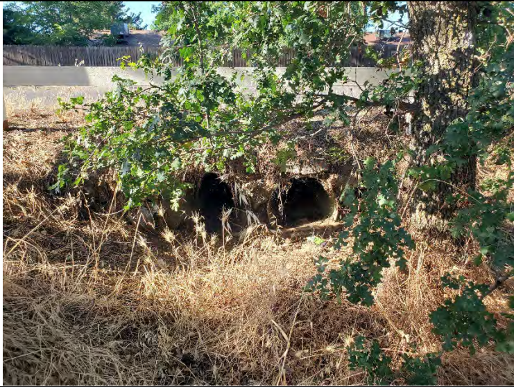
Facing south, culvert on Main Street.
